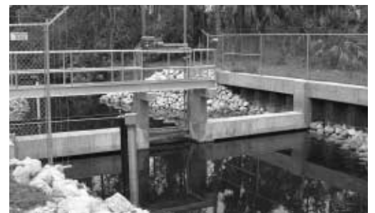
Water Control Structure
